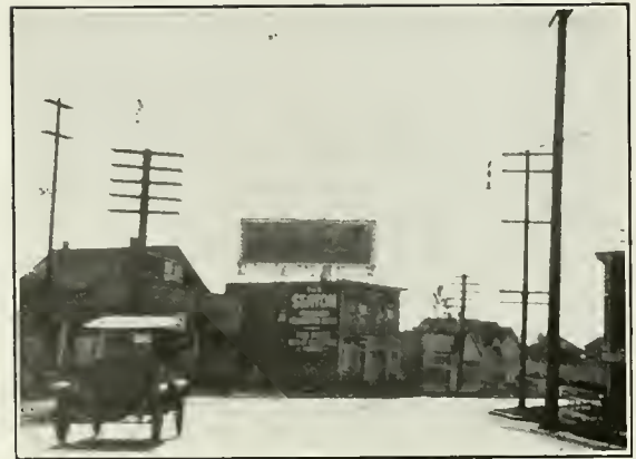
Bad Curve on Kingsway at Tyne Street Should be Rectified. Looking North-West.
