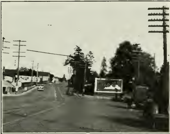
Kingsway at Knight Street will Require Widening. Looking South-East.
