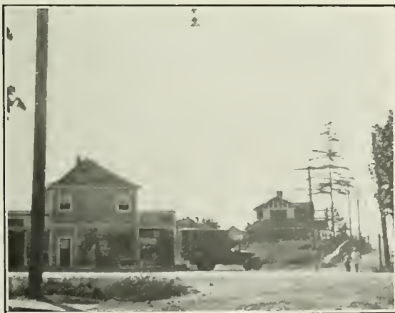
School Road at Joyce Road Where Forty-first Avenue will Emerge. Looking West.
