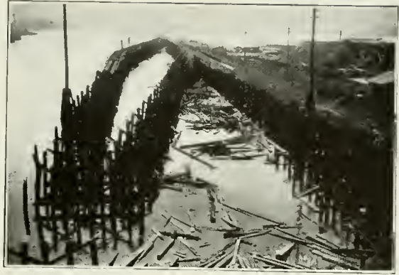
False Creek. An Example of Conditions in This Area Which Require Cleaning Up.
