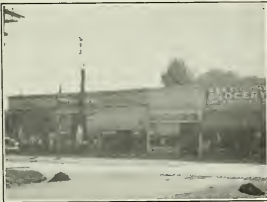
Frame Buildings to be Removed for Elimination of Jog at Forty-First Avenue and Victoria Drive. Looking West Across Victoria Drive.
