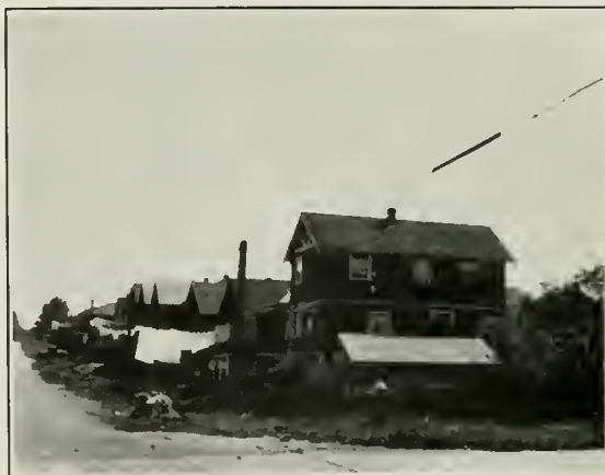
Rear View. Along Prince Edward Street.
