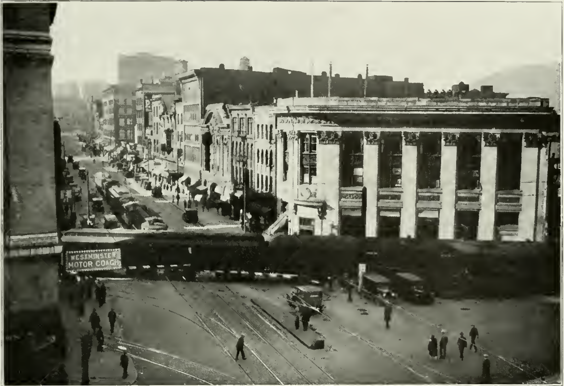
C.P.R. Carrall Street Level Crossing.
