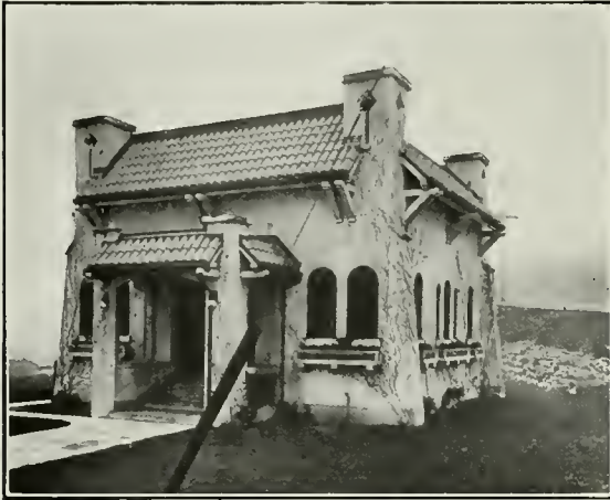
An Appropriately Designed Transformer House in a Residential Neighbourhood.
