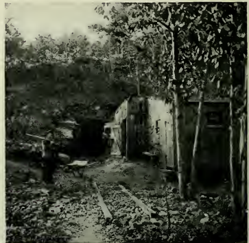
THE MOUTH OF THE TUNNEL
