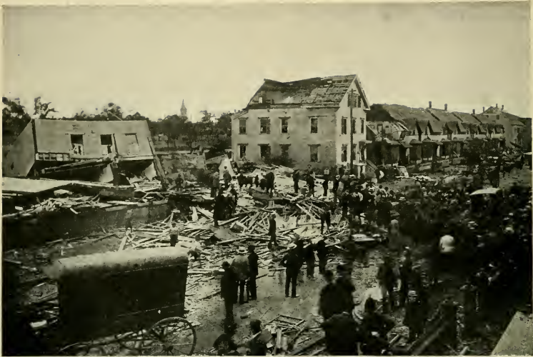
AT THE END OF SPRINGFIELD STREET, SHOWING HOUSE MADE ROOFLESS AND TURNED OVER
