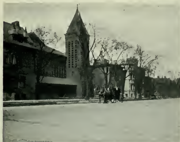
JEFFERSON AVE. PRESBYTERIAN CHURCH
