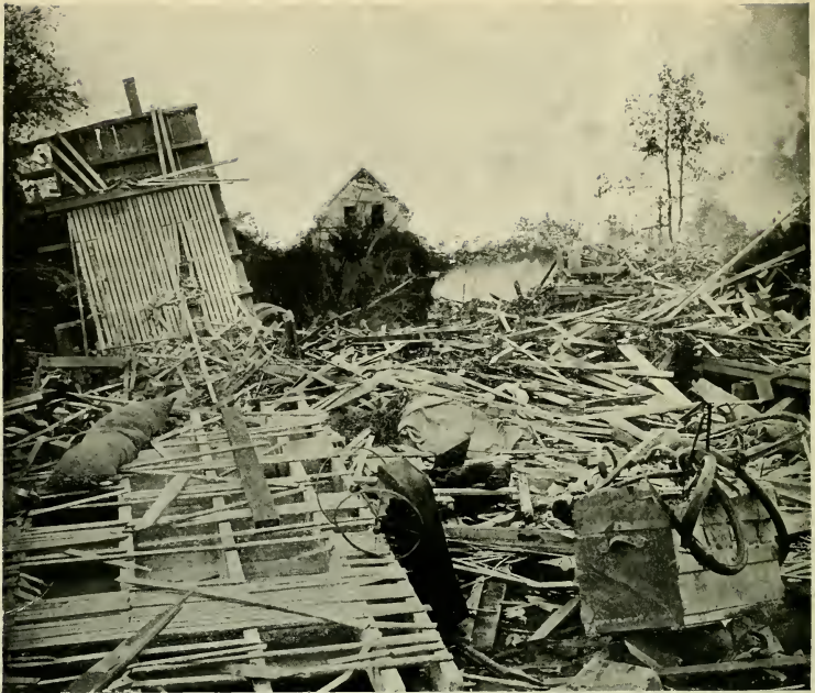
THE LOWELL DISASTER — THE RIGGS HOUSE, COMPLETELY DEMOLISHED
