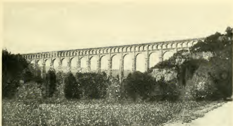
ROQUEFAVOUR AQUEDUCT, MARSEILLES CANAL
