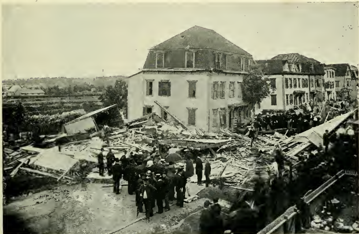
SPRINGFIELD STREET, NEAR THE CORNER OF FOSTER, SHOWING HOUSES COMPLETELY DEMOLISHED, WHILE OTHERS NEXT TO THEM ARE UNINJURED
