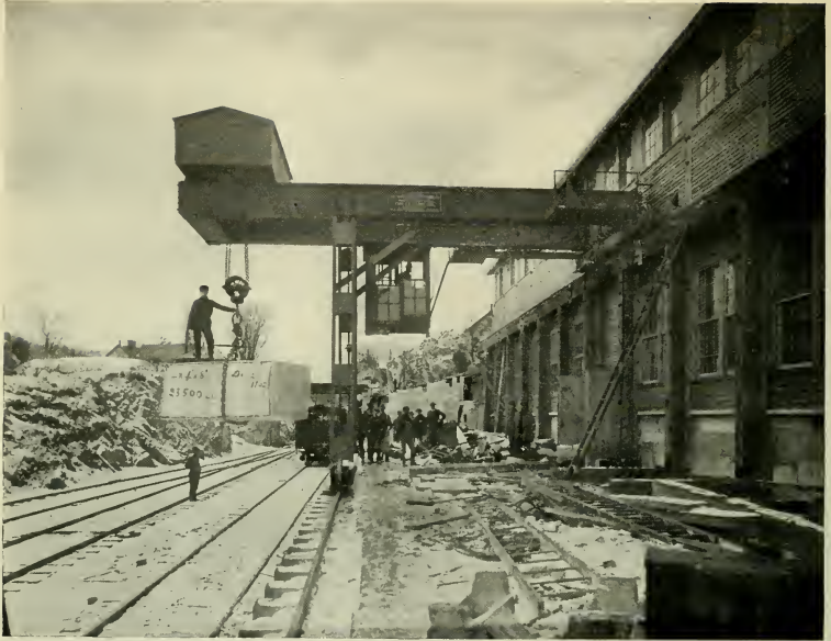
LOADING A TWELVE-TON BLOCK, PROCTOR
