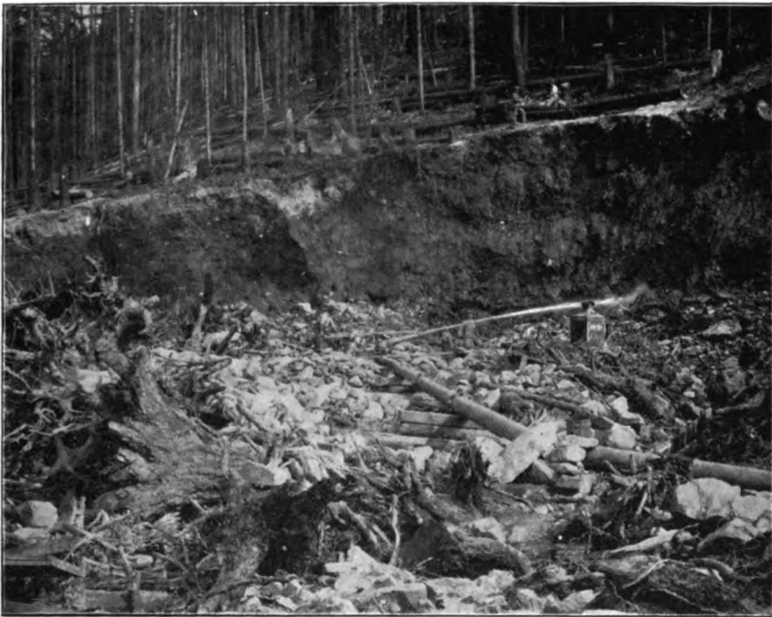
FIG 54.—NORTHERN PACIFIC RAILWAY, HYDRAULIC-FILL CONSTRUCTION. VIEW IN PIT SHOWING HYDRAULIC GIANT IN ACTION.
