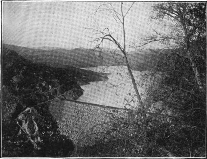
FIG. 10a.—ESCONDIDO (CAL.) ROCK-FILL DAM. WOODEN LINING. [To face page 18.]
