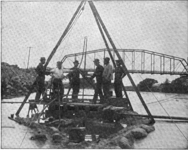
FIG. 153.—BORING APPARATUS, CONSISTING OF PILE-DRIVER AND DIAMOND-CORE DRILL AT WORK. USED FOR TESTING BED-ROCK AT GILA RIVER DAM-SITES, ARIZONA.
