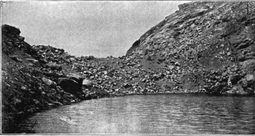
FIG. 19.—MORENA ROCK FILL DAM IN PROCESS OF CONSTRUCTION. SHOWING TOP OF TOE-WALL ABOVE THE WATER-LINE.
