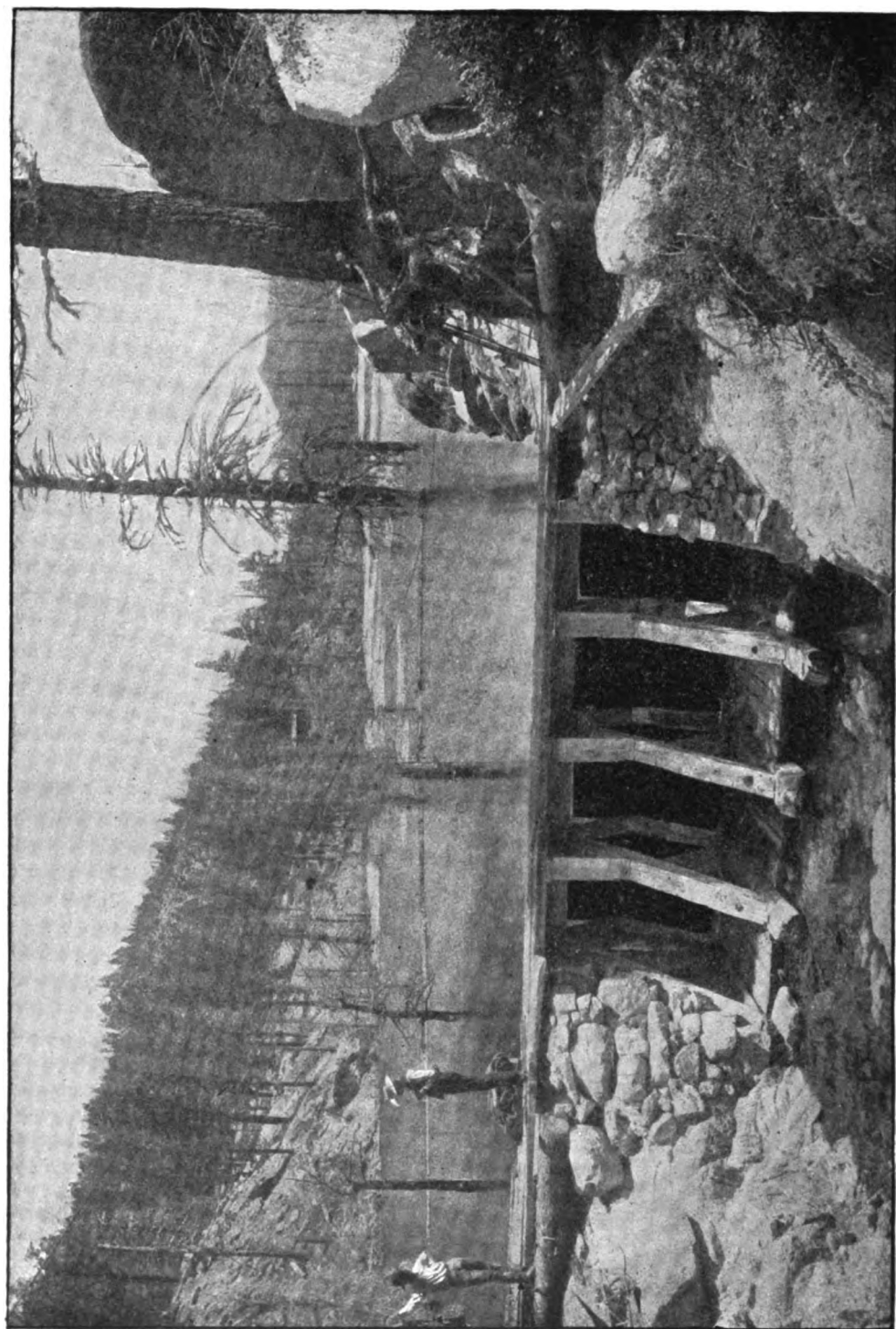
FIG. 80.—SPILLWAY OF BEAR VALLEY DAM, WITH FLASHBOARD GATES.
