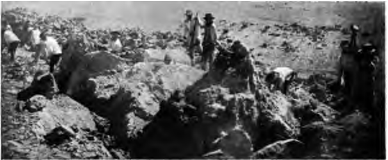
The Nitrate Pampa: Opening up Trench after Blasting.
