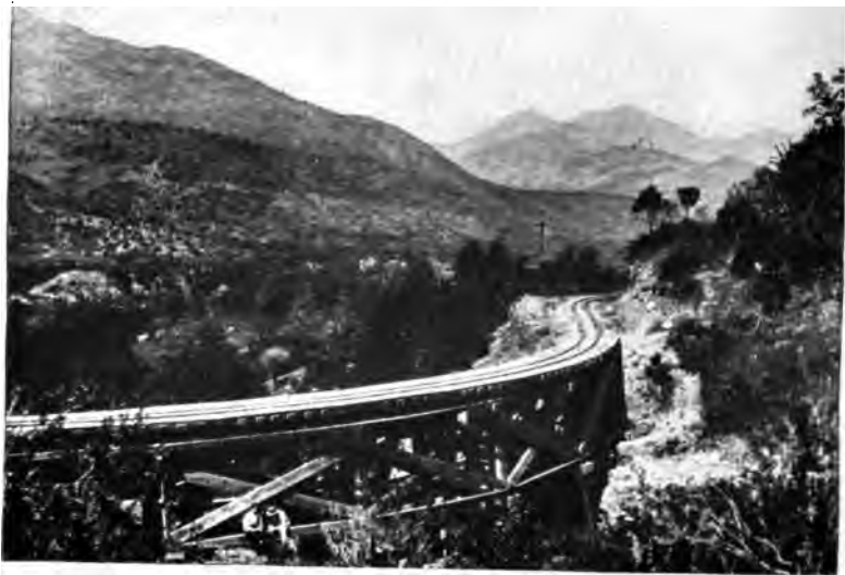
Railway between Rancagua and El Teniente.
