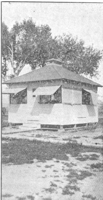
BUNGALOW, EAST FARM SANATORIUM.
