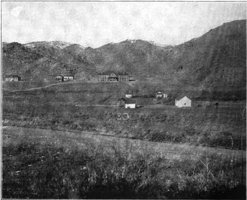
TRUXTON CANYON SCHOOL, ARIZONA.
