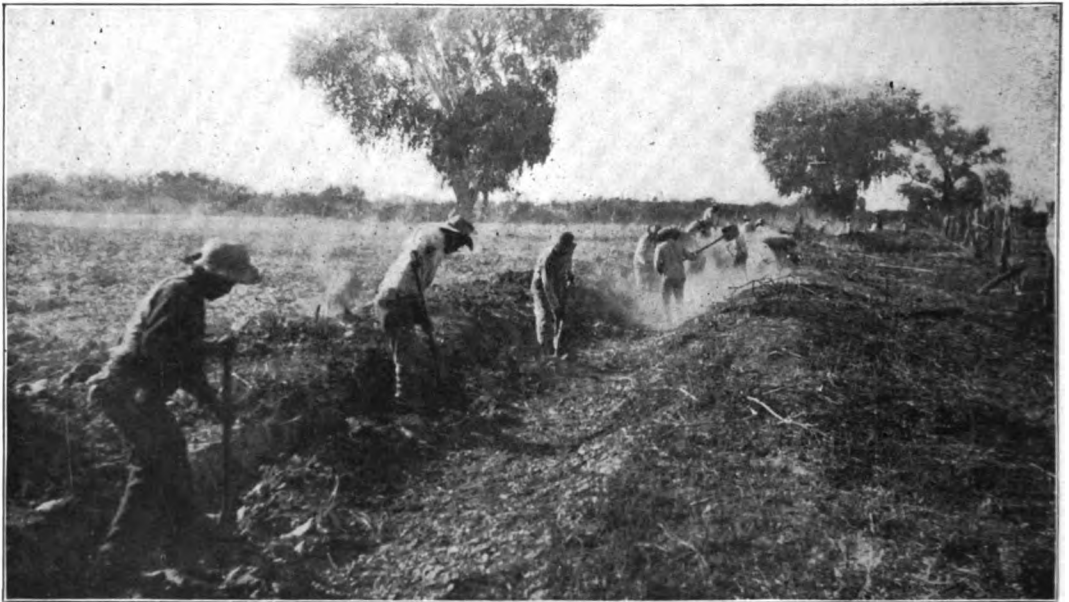
PIMA CLEARING OUT THEIR DITCHES AT BLACKWATER, ARIZONA.
