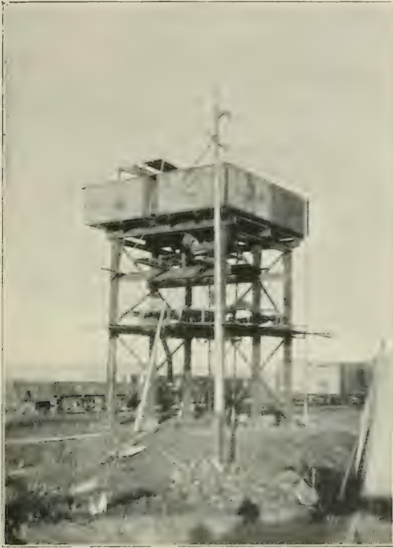
“PERCHED ON THE TOP OF WATER-TANKS.”
