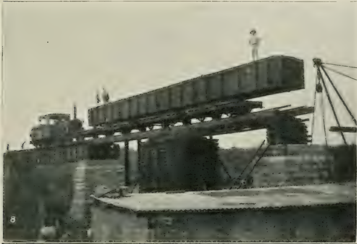
“THE GIRDER WAS RUN OVER ITS EXACT PLACE.”
