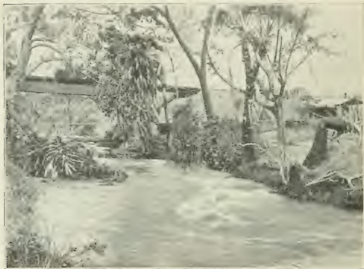
“THE RIVER CROSSED BY MEANS OF A TEMPORARY BRIDGE.”
